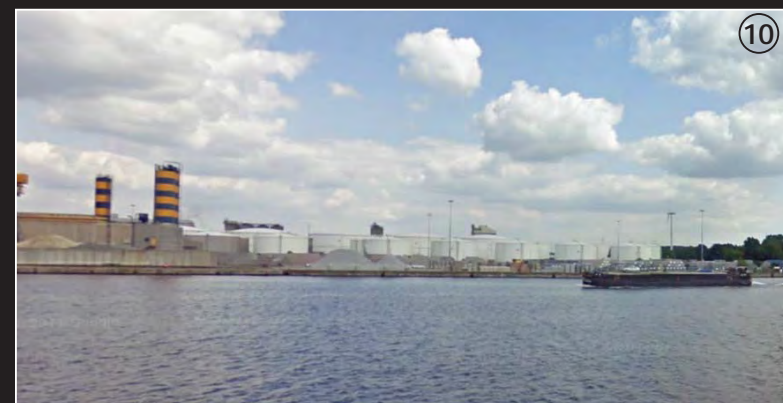
Tanks van Oiltanking
