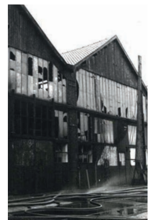
Gevel na brand in 1964
